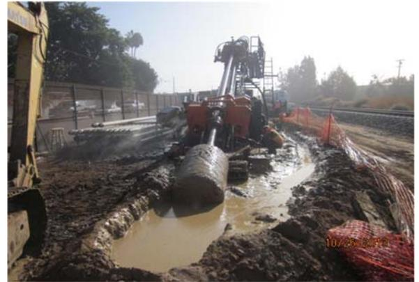
*SGTC Fiber Optic Installation Drilling*
