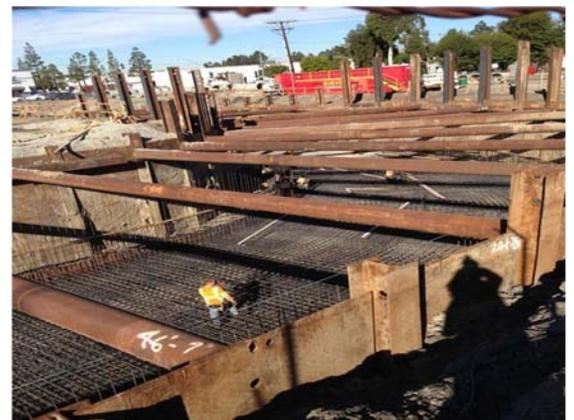
*Nogales Storm Drain Line A Rebar for Concrete Floor*
