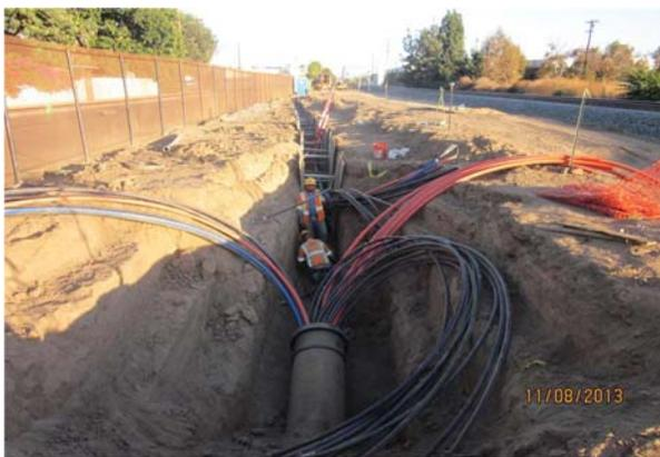
*SGT Fiber Optic Cable Pulling and Splicing*
